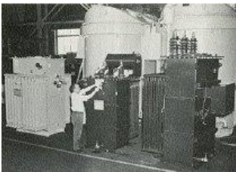
Part of the power transformer shipment destined for the Snowy Mountains Hydro-Electric Project in Australia. It included 16 units of 68,000 Kva, 345,000 volts. GE Pamphlet, Guelph Museums
